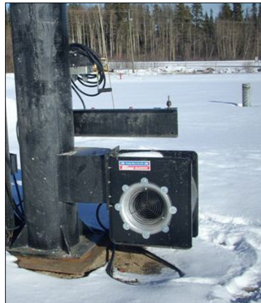
Figure 1: Some flare stacks contain a fan at the base that induces extra atmospheric air, producing greater combustion and making the flare a more efficient burn, which results in fewer emissions to the atmosphere.
