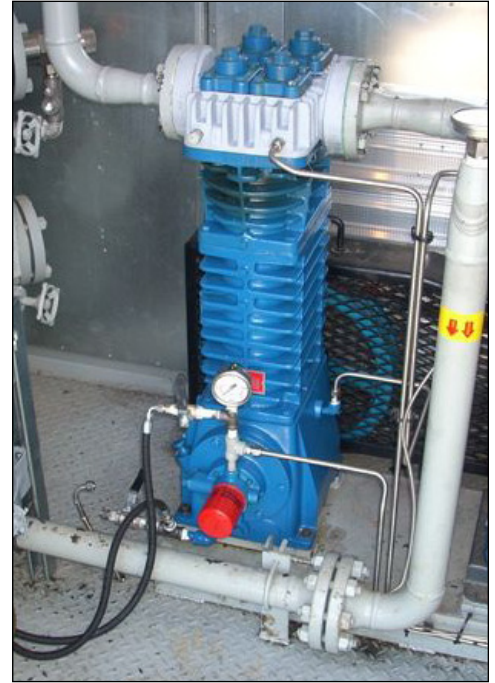
Figure 6: Vapour Recovery Unit (VRU): A unit composed of a scrubber, a compressor and a switch. The VRU's main purpose is to recover and condense vapours formed inside tanks. The switch detects pressure variations, in turn switching the compressor on and off. Vapours are drawn through the scrubber, where the liquid is trapped and returned to the liquid pipelines system or the tank, and the vapour recovered is pumped into gas lines.
